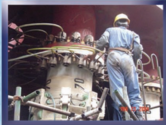
Hydraulic Bolt Tensioning
