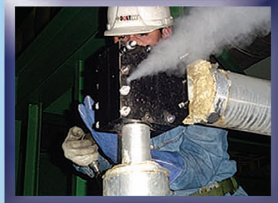
On-Line Leak Sealing
